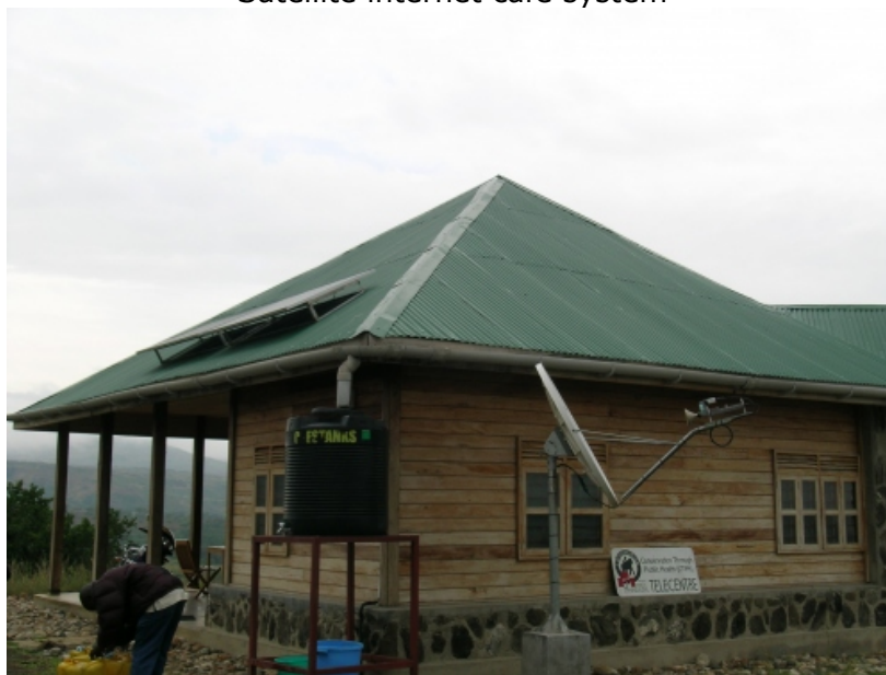
PV array, rainwater catchment, VSAT dish
